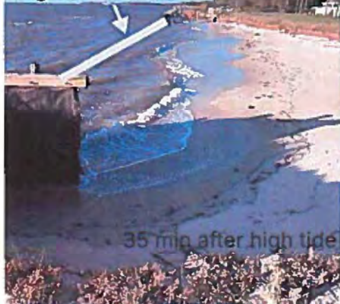
Approx location of original revetment
